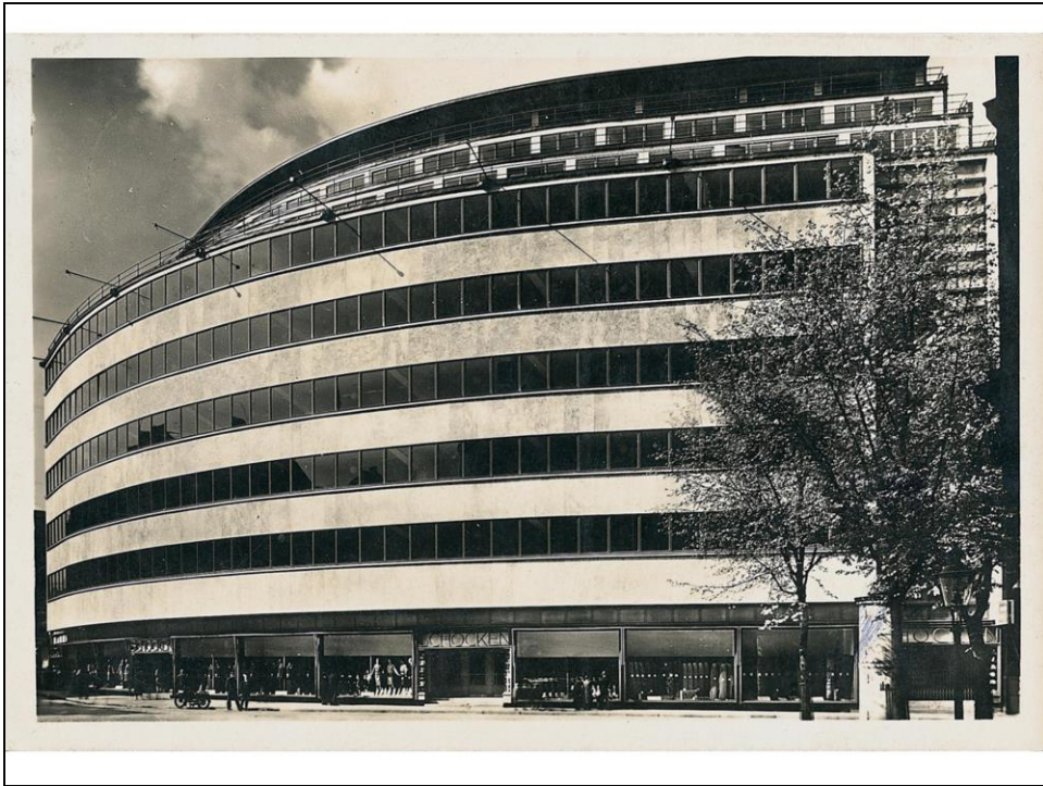
E. Mendelsohn, Grandi Magazzini Schocken, Chemnitz (1926-28)
