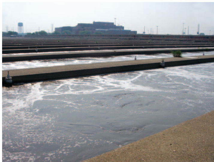
FIGURE 3 Aeration basin for activated-sludge processing at a large metropolitan wastewater treatment plant, Stickney, Illinois. PHOTO: REIKA YOKOCHI
