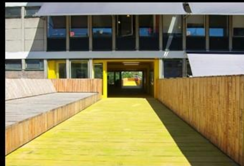
Luchtsingel pedestrian footbridge
