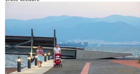
Several cascading thermo-wood surfaces installed on a steel frame allow users to enjoy the view of the bay.
