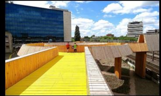
Center of the Bridge
