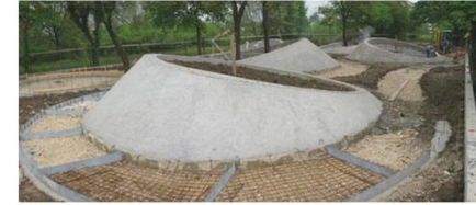
Pic of construction phase
