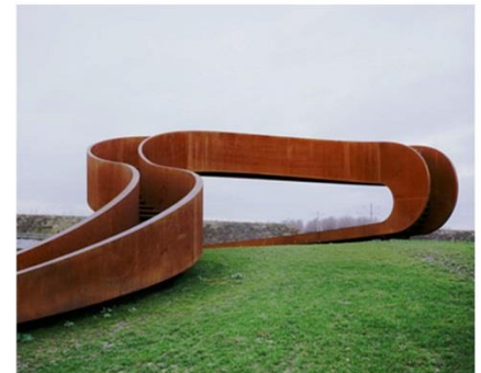
The design is based on the principle of a Möbius Strip, and it is built from pre-weathered corten steel, giving it a vivid orange tone that contrasts with the bright green of the grass below.
