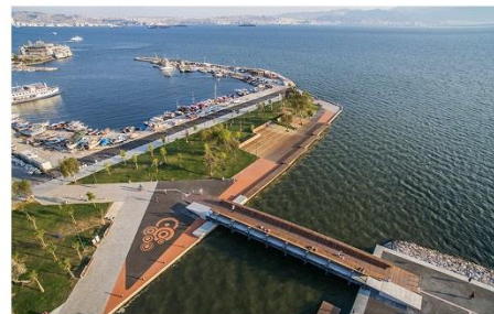
The footbridge connects the two sides of bostanlı creek.
