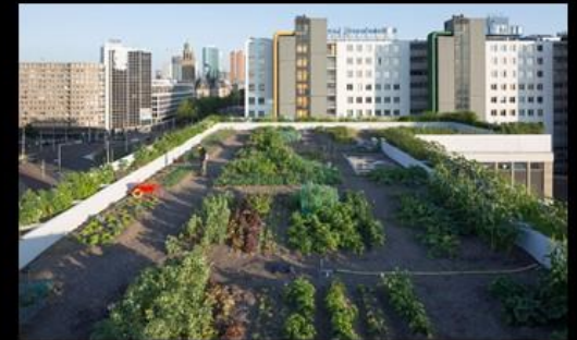
DakAkker Roof Garden on the Schieblock Building
