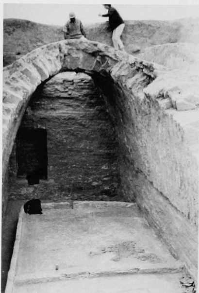
B. Vaulted Tomb of Tepti Ahar: south end of tomb chamber showing passage to Hall no. 1, remaining vault, and burial platform in B XX.
