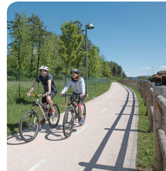
Cycle path made with permeable paving, Calusco, Bergamo, Italy. (i.idro DRAIN by Italcementi S.p.A. – photo Italcementi).
