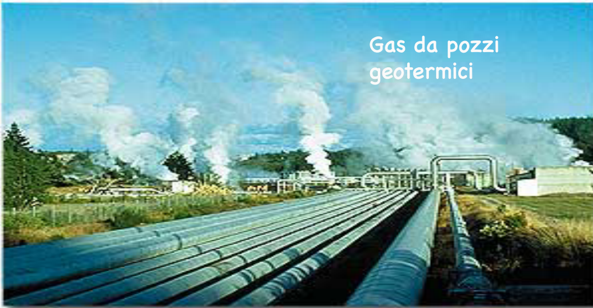
Steam pipelines, Wairakei Power Station
