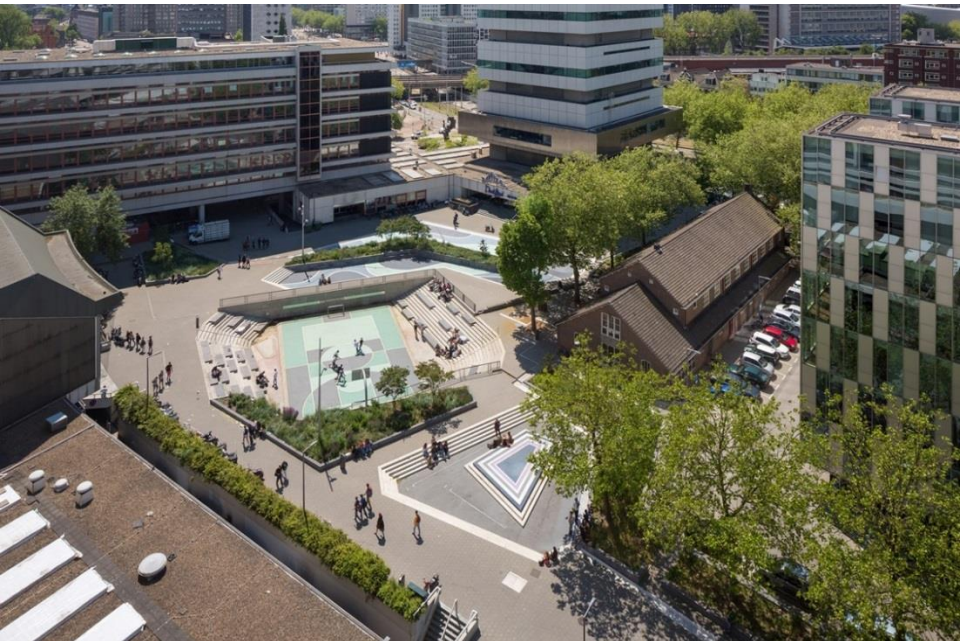
Water Square, Rotterdam The Netherlands © De Urbanisten
