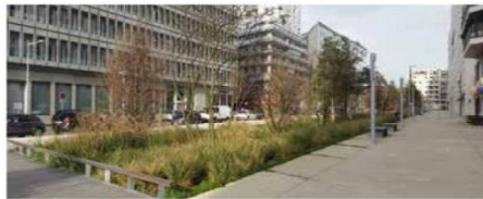
Parc de Billancourt, Paris, AGENCE TER, 2011. Un bioretention swale lungo Avenue Emile Zola a margine del parco testimonia il perfetto connubio tra WSUD e architettura del paesaggio / A bioretention swale on the Avenue Emile Zola on the edge of the park reveals the potential combination of WSUD and landscape architecture (© Lucio Lorenzo Pettine)
