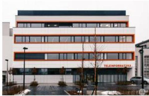
Department of Telecommunications, II
