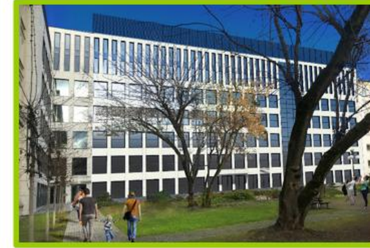
Construction of a new teaching facility for the Faculty of Humanities, the Faculty of Applied Mathematics, the Department of Foreign Languages
