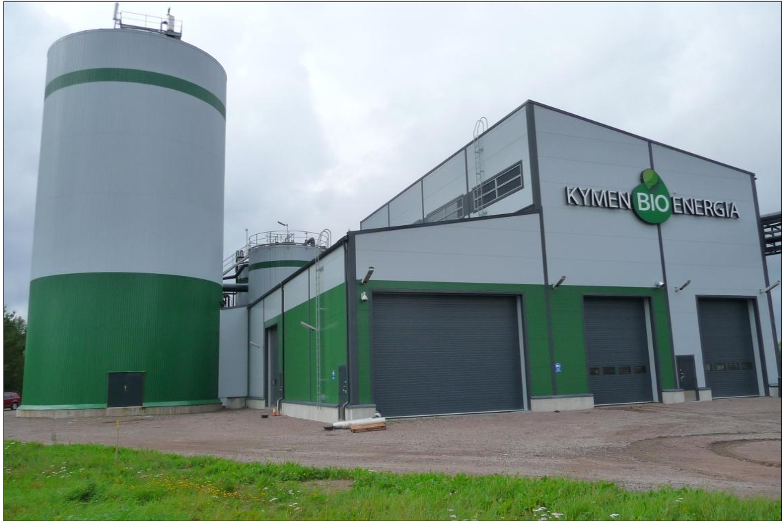
Figure 8. Anaerobic digester for all wet organic waste from city of 90,000 in Finland – approximately 80,000 m 3 per year of 10% dry matter.
