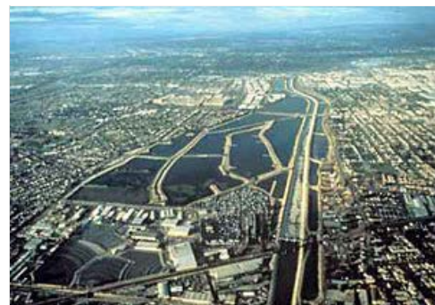
For over 35 years, in the Montebello Forebay Ground Water Recharge Project, recycled water has been applied to the Rio Hondo spreading grounds to recharge a potable ground water aquifer in south-central Los Angeles County.
