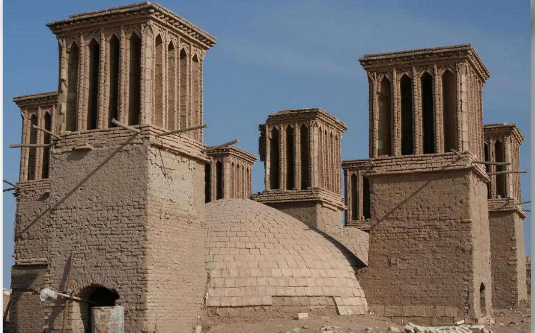
Bevels were incorporated to reduce turbulence and enhance wind capture
