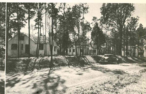
A group of houses on Pine Road including (left) a five-room house (Type 54) and four-room houses (Type 41). A primary consideration was to take advantage of good sites without felling trees
