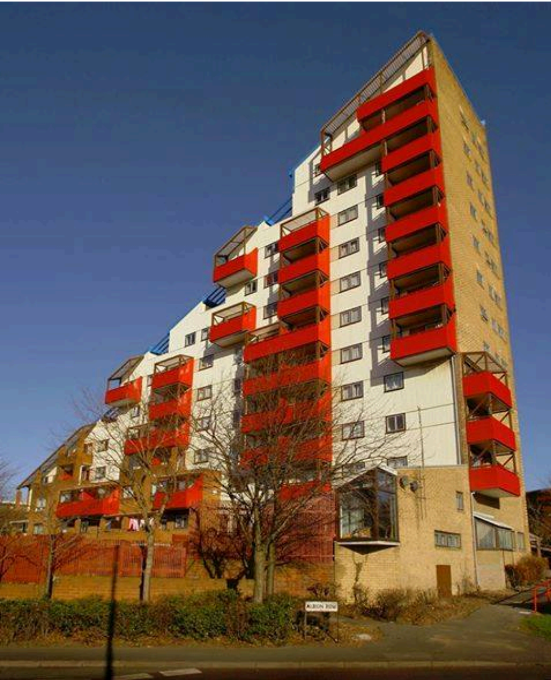
Newcastle-upon-Tyne - Byker Wall, Inghilterra
