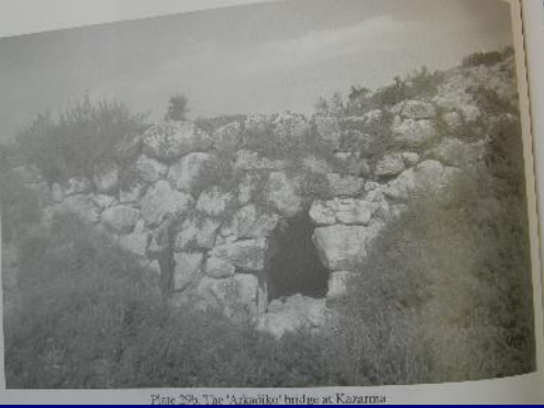
Plate 29b The 'Arzaviko' bridge at Kazarma
