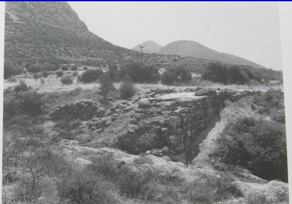
Fig. 18. Bridge across Khavos and revetment wall.
